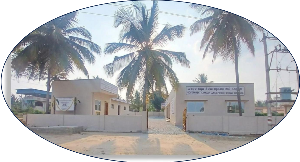
Government School & Anganwadi building construction
